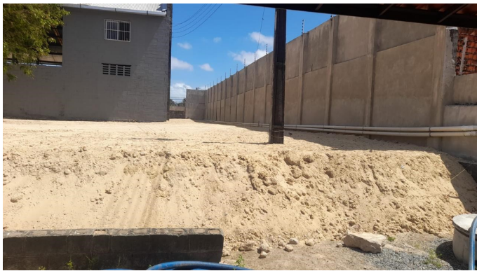
54 lorries of sand to help level the ground
